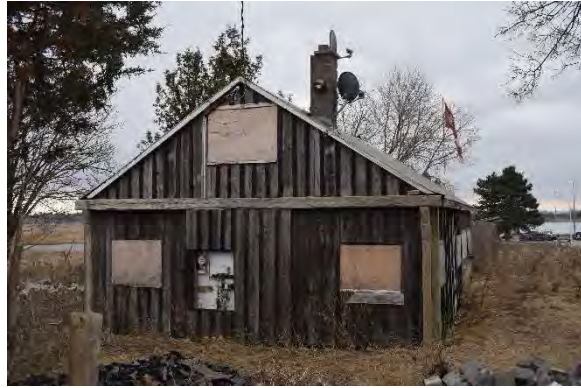
Photo 47: North façade, looking south
