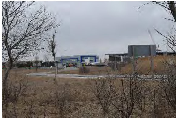
Photo 4: Highway 400 offramp, looking west
