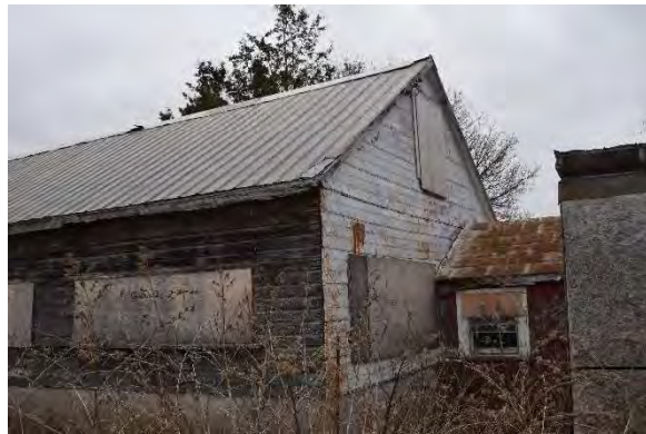
Photo 49: South façade, looking east
