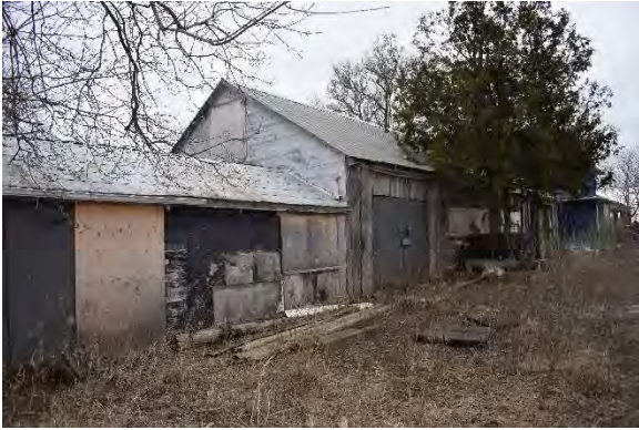
Photo 46: Secondary entrances, looking north
