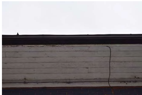
Photo 14: Representative photo of roof soffit
