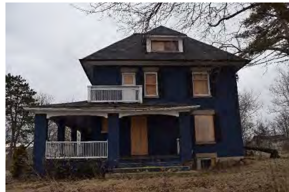
Photo 16: Front façade, looking south
