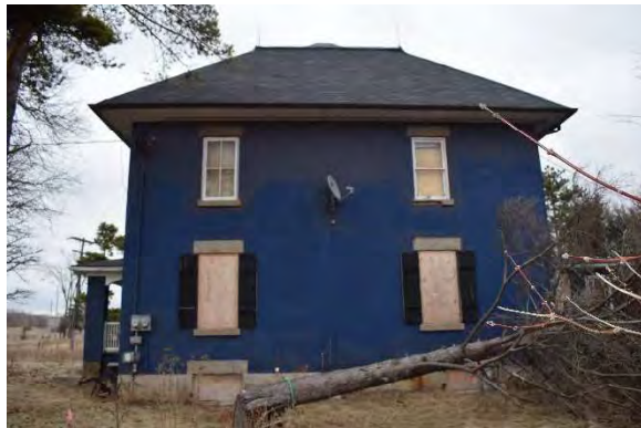
Photo 28: West façade, looking east
