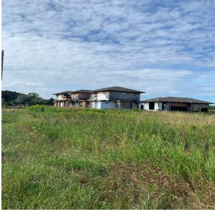
Photo 1: View of abandoned residential properties at intersection of Dale Crescent and Line 13, facing southwest.
