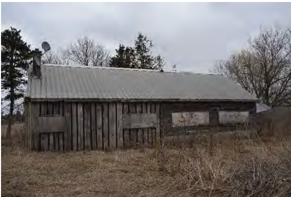
Photo 48: West façade, looking east
