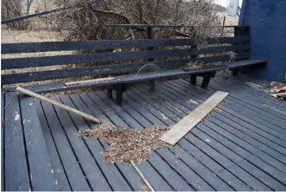
Photo 35: Deck, looking west
