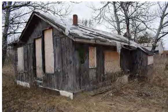
Photo 51: Southwest outbuilding, looking east
