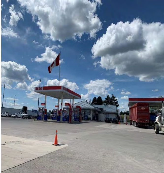
Photo 11: View of Esso/ Bradford Husky gasoline service station for both trucks and regular sized vehicles, facing west.
