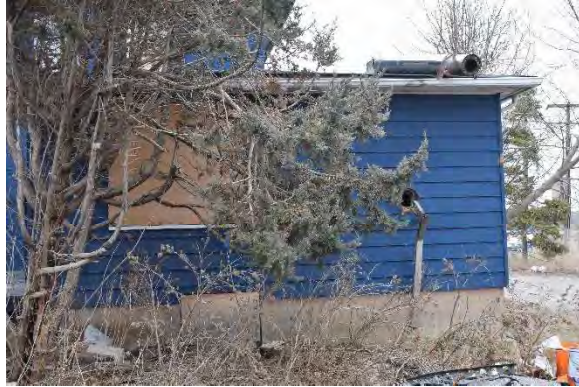
Photo 36: South façade of addition, looking north
