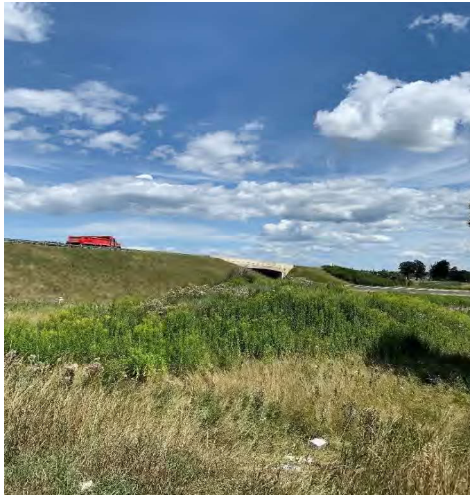
Photo 9: View of berms and bridge at junction of County Road 88 and Highway 400, facing west.
