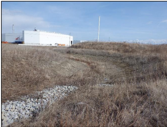
Figure 8: Widened channel corridor is confined by graded berms close to Crossing 2 (Figure 1) at 10 Sideroad.
