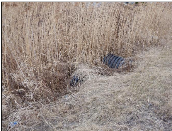
Figure 4: Dual Culvert outlet into phragmites lined swale.
