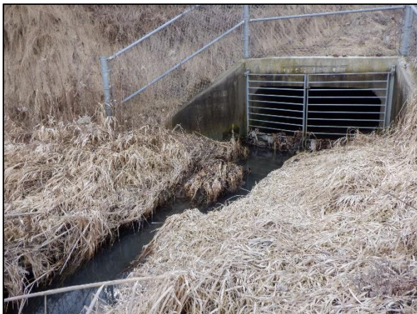
Figure 12: Box Culvert at Crossing 4 (Figure 1) on the North side of Line 8.
