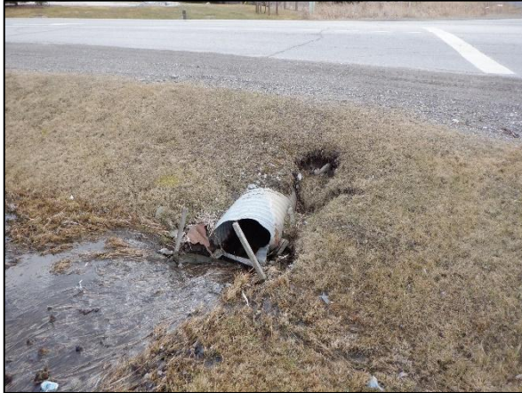
Figure 6: Bank erosion on the northeast corner of Line 8 and 10 Sideroad.
