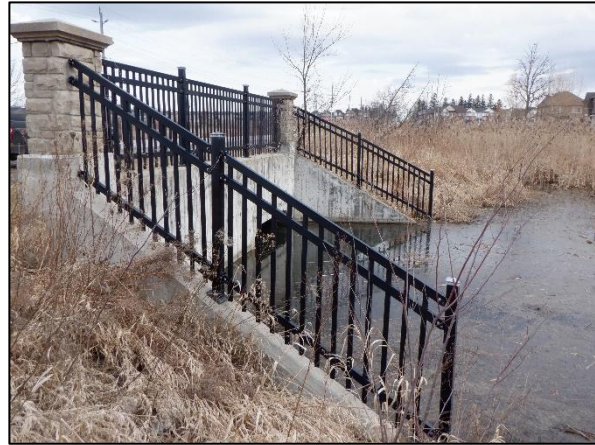
Figure 11: Twin concrete box culverts outlet to a wetland on the south side of Line 8 at Crossing 3 (Figure 1).
