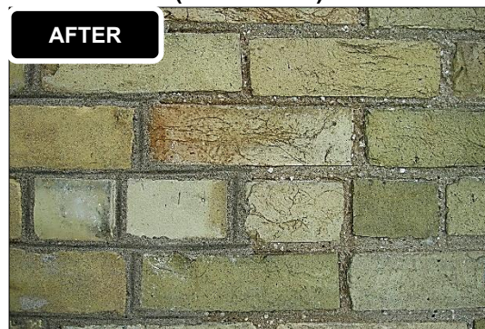
New lime rich mortar is applied to the joints. Repointing work is complete. (Source: GDV)
