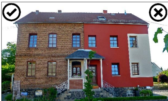
An extreme example of over cladding where the right side of the brick masonry façade is covered with EIFS (Source: Handwerker)
