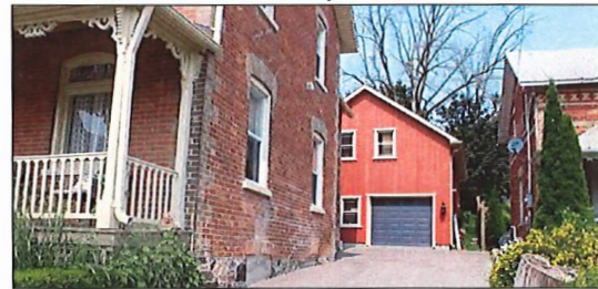
4334 County Rd. 88 – stand-alone garage structure located at the rear of the property (Source: GDV)
