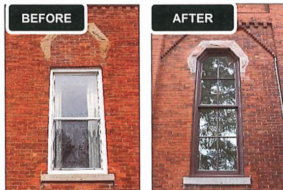
Example of window restoration / replacement based on historic document of originals. (Source: GDV)
