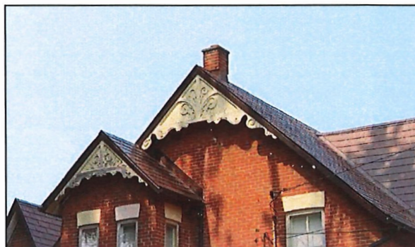
2870 County Rd. 27 – Gable details (Source: GDV)
