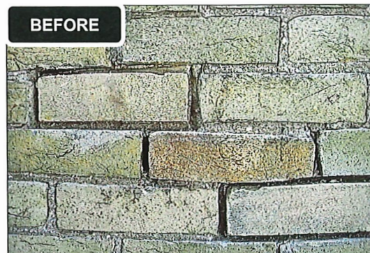
Deteriorated mortar joints require repointing. Deteriorated joints are cut-out using handheld tools prior to repointing. (Source: GDV)
