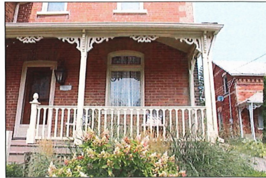
4334 County Rd. 88 – front porch (Source: GDV)
