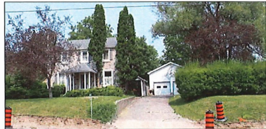
4354 Line 7 – stand-alone garage structure located at the rear of the property (Source: GDV)
