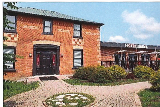
4240 County Rd. 88 – outdoor pathways (Source: GDV)
