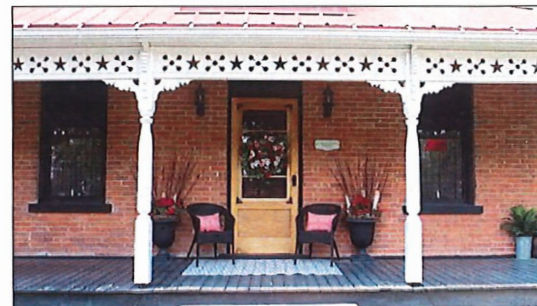
70 Hearn St. – Verandah (Source: GDV)
