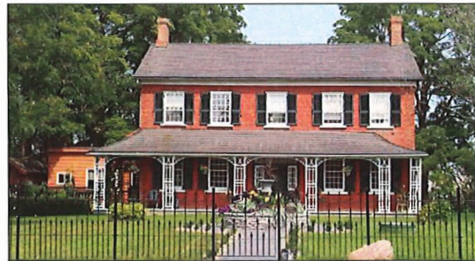
4370 Line 7 – Verandah (Source: GDV)
