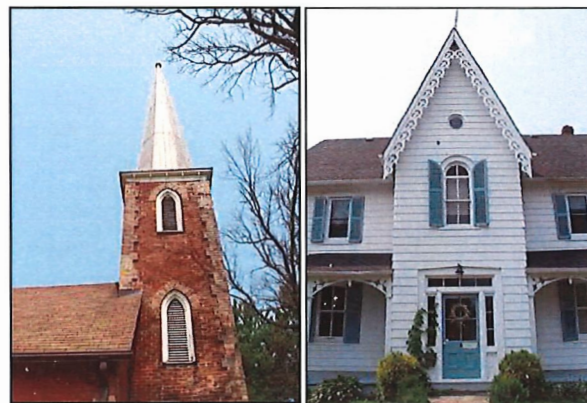
56 Hearn St. (left) and 2876 County Rd. 27 (right) (Source: GDV)
