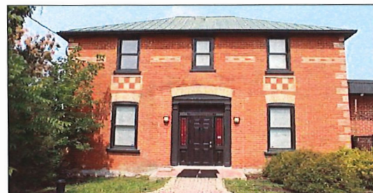
4240 County Rd. 88 – entrance door with sidelights and transom (Source: GDV)
