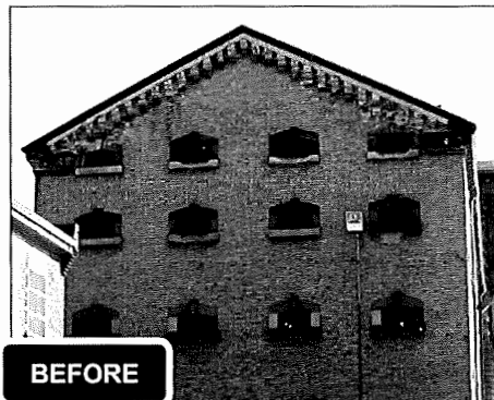
Example of heritage masonry façade prior to cleaning (Source: GDV)
