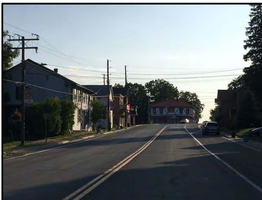
Image 11: View 2 – Terminating Short-View to Brazill House (Hotel) West Down CR 88 (August 1, 2019; View Facing West)
