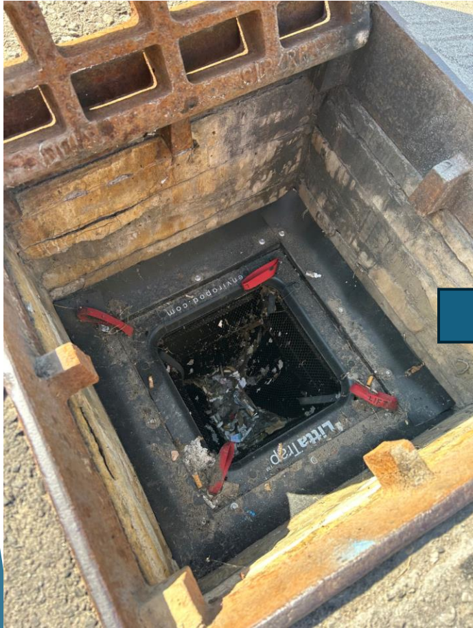
Figure 5: LittaTrap collecting waste
