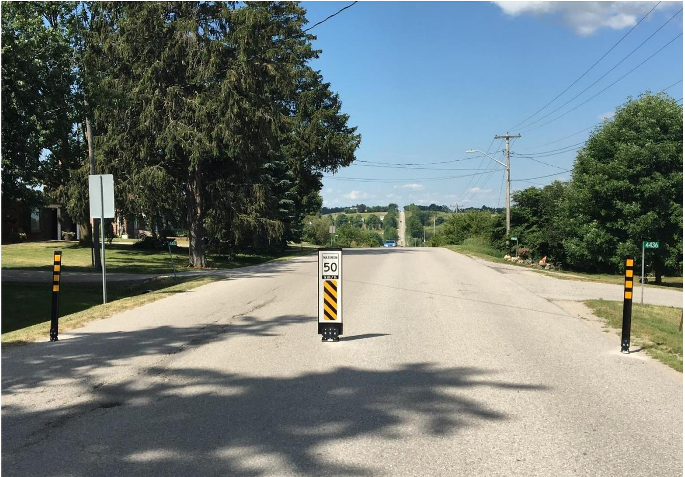
*Traffic bollards installed in locations including this one on Line 7 in Bond Head will remind drivers of the posted speed limit while giving the impression of a narrower road, encouraging them to slow down.*
