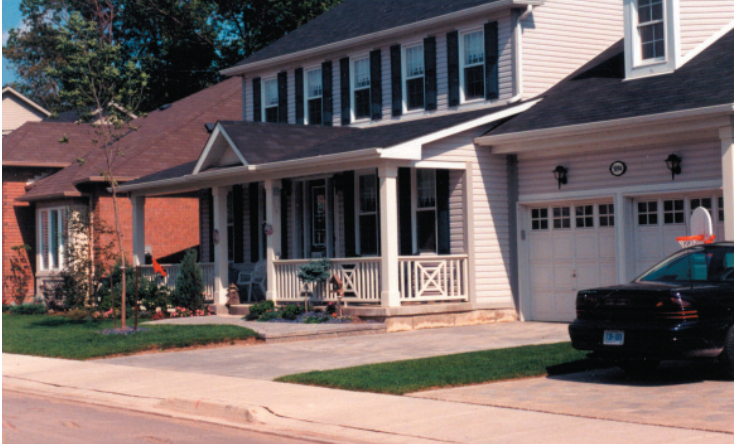
Photo 11: Housing should be designed to project a strong public face, though the inclusion of front porches, rooms that face the street and garage setbacks
