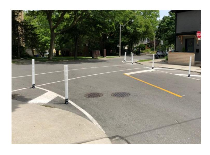
Use paint markings to signal changes in speed and pedestrian presence to drivers
