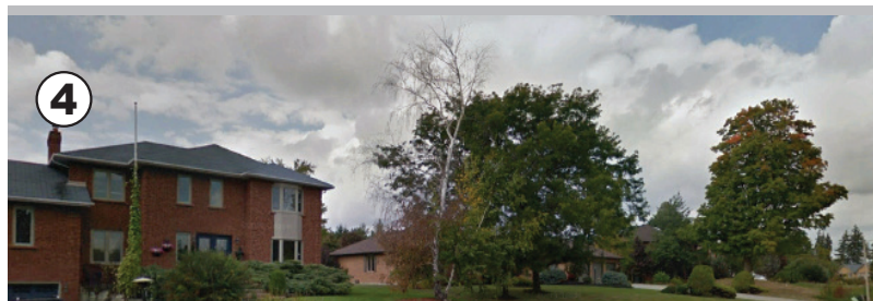
Views of existing residential on Brownlee Drive
