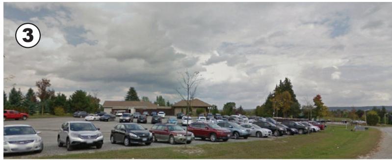
View of the clubhouse and parking area associated with the former Bradford Highlands Golf Club from Brownlee Drive.
