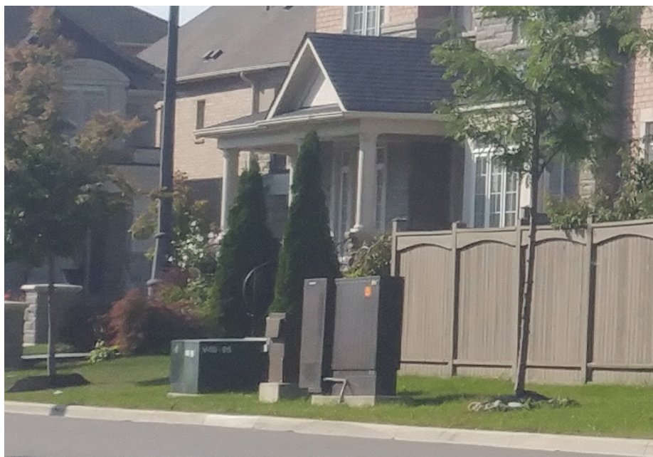
Example of grouped utilities within the streetscape
