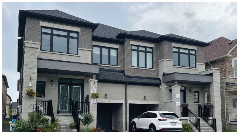
Promoting architectural variety, innovation and quality with complementary landscape and open space features
